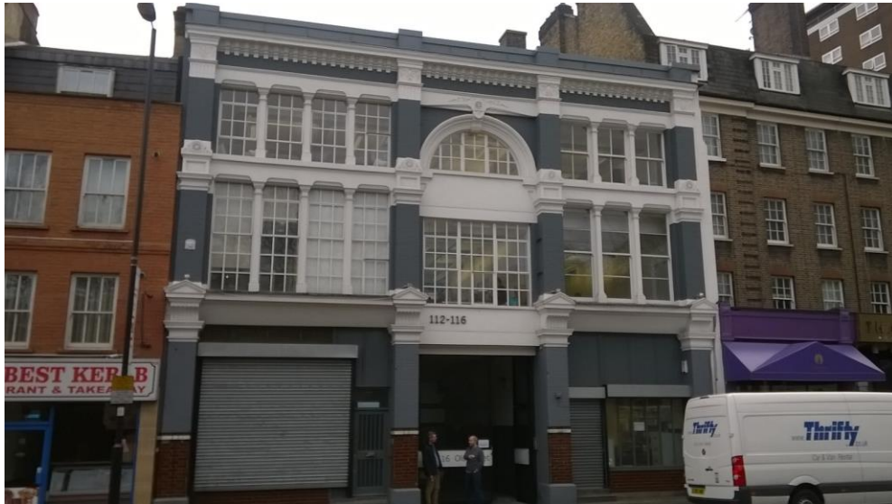
View of building frontage from Old Street
