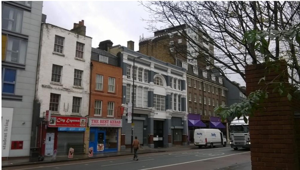
View of site looking south-west
